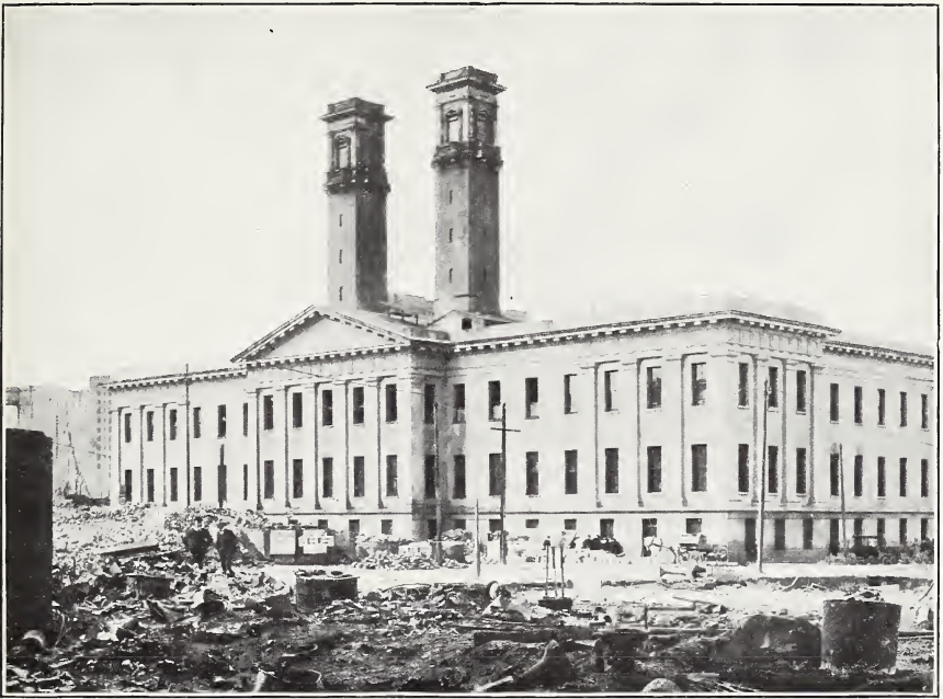
A. GOOD EARTHQUAKE ENDURANCE OF A BUILDING OF THE MONUMENTAL TYPE: UNITED STATES MINT, SAN FRANCISCO.
